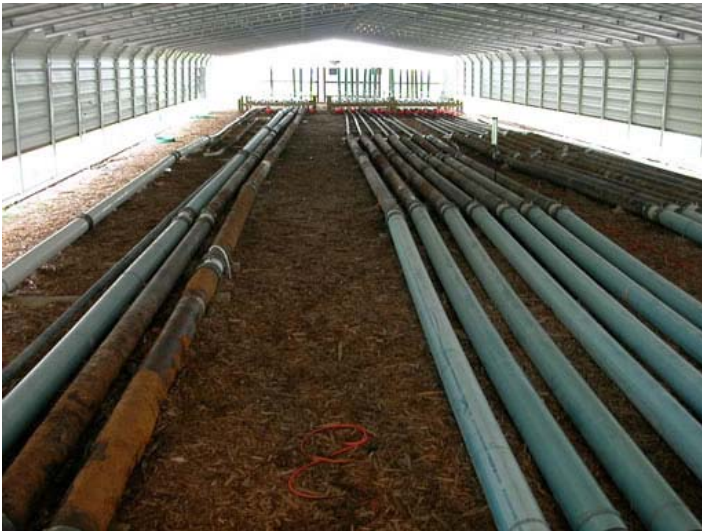
Figure 2 Distribution System of Pilot Plant
